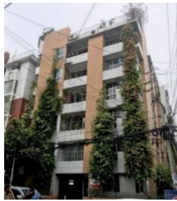
Figure 2: indirect green facade with Bougainvillea plant
